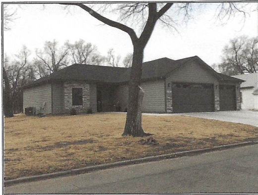
433 W. Fourth, Solomon, Kansas 3 bedroom, 2 bath home, 3-car attached garage on slab. Dilapidated structure & numerous trees removed, dirt hailed in for "pad", electricity brought in to lot Constructed & sold for approximate $32,500.00 loss.
