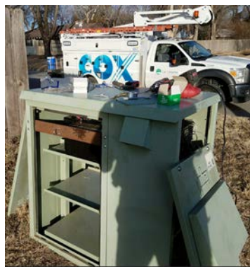
With Security bar installed
