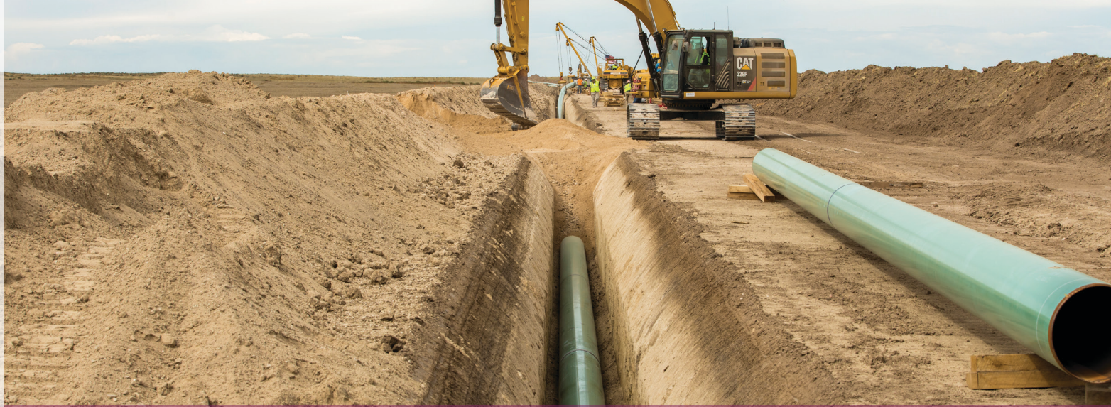
Construction on the Elk Creek Pipeline
