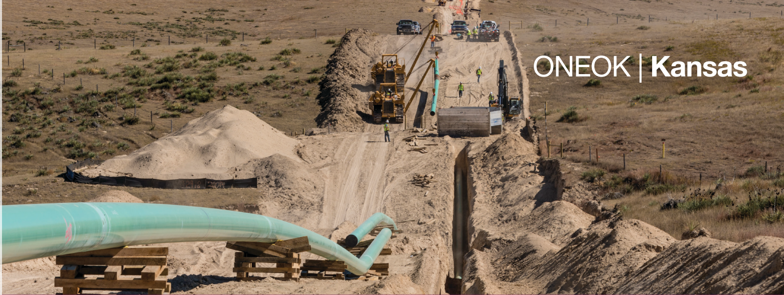
Construction on the Elk Creek Pipeline
