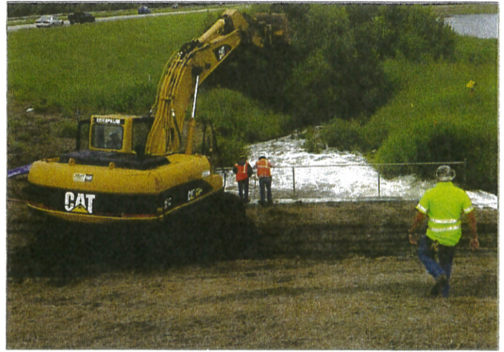
ABOVE: Corps Levee Project – 500-yr Flood Protection
