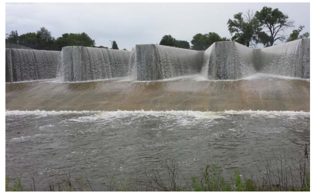
ABOVE: Augusta City Lake Spillway/Dam Project
