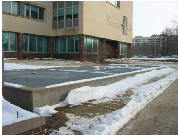
Photograph 3: South Side of DSOB Areaway
