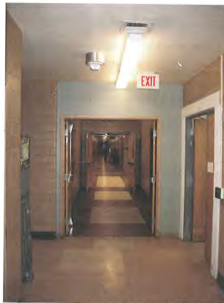
Photograph 10: North-South Hallway, Basement Level, Looking North
