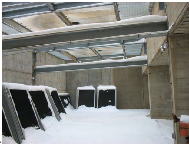
Photograph 4: DSOB South Areaway
