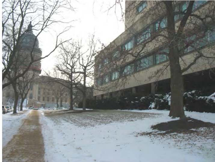
Photograph 1: North Side Docking State Office Building
