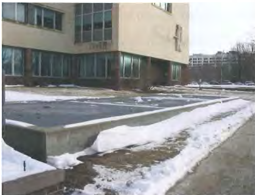
Photograph 5: South Side of DSOB Areaway
