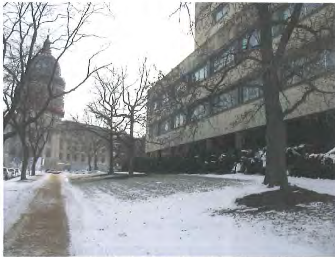
Photograph 3: North Side Docking State Office Building
