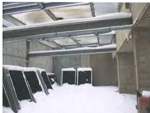
Photograph 6: DSOB South Areaway
