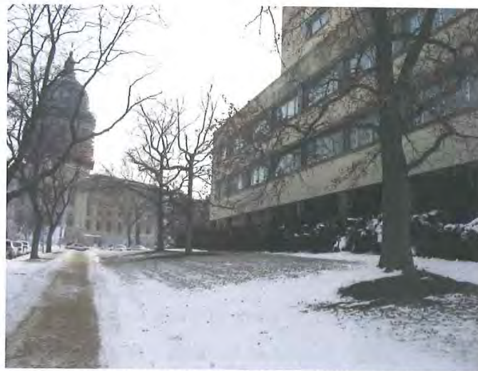
Photograph 7: North Side Docking State Office Building
