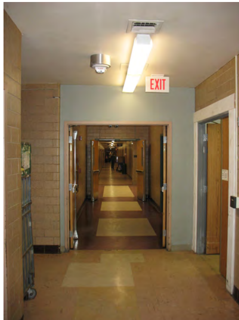
Photograph 5: DSOB South Arealway
