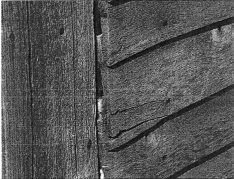
View of split wood siding
