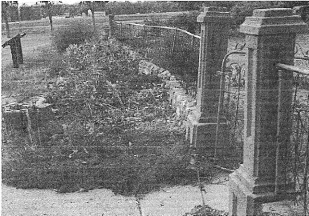
View showing base of tree pushing over stone fence and concrete post
