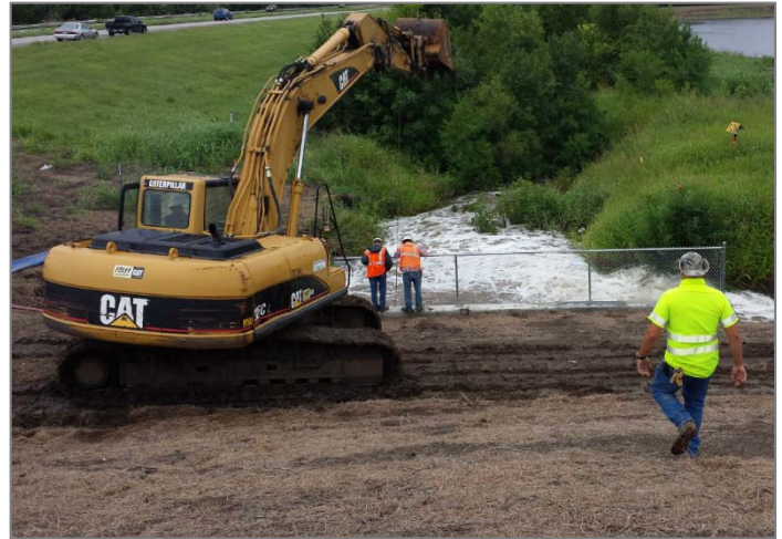
ABOVE: Corps Levee Project – 500-yr Flood Protection
