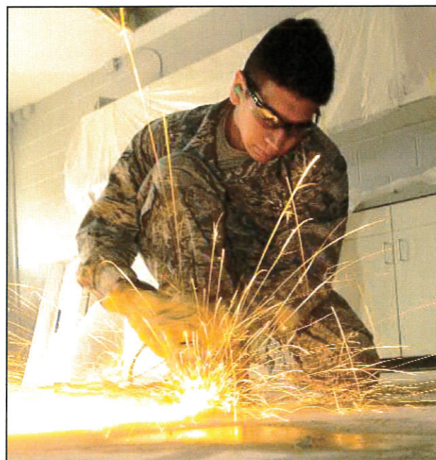
Airman 1st Class Edgar Maldonado, 184th Civil Engineer Squadron, cuts an anchor bolt from the Ottawa Armory floor after removing an 8-inch concrete masonry unit wall.
