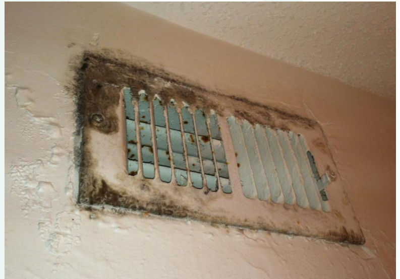
Mold on ceiling vent:
