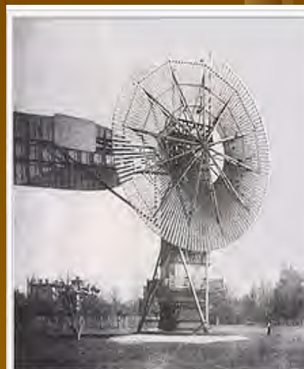
The first automatically operated wind turbine, built in Cleveland in 1887 by Charles F. Brush. It was 60 feet (18 m) tall, weighed 4 tons (3.6 metric tonnes) and powered a 12kW generator. [17]
