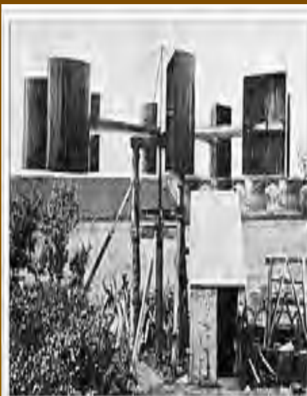
James Blyth's electricity generating wind turbine photographed in 1891
