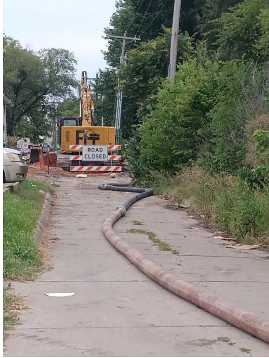
Above shows day work just starting on Sewer line on 8/9/2024
