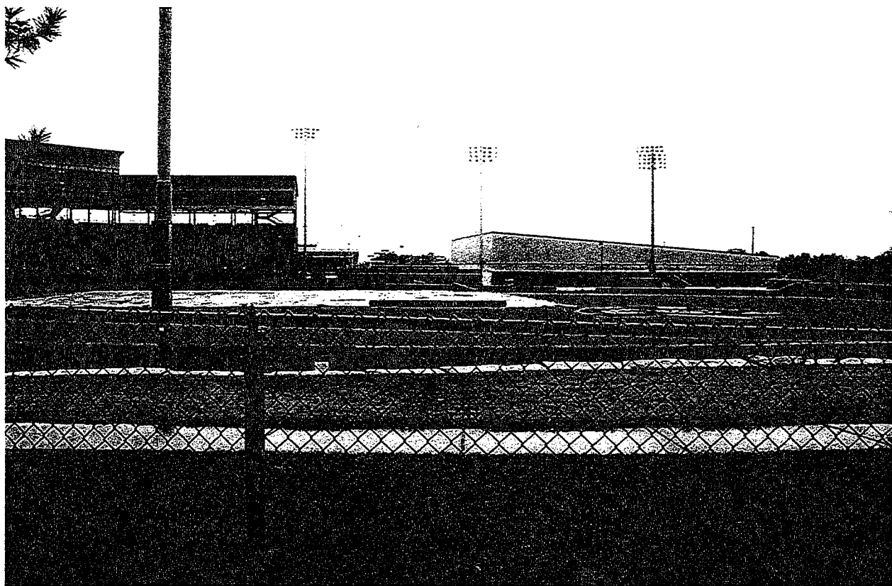
Exterior / Bombardier Learjet Practice Facility
