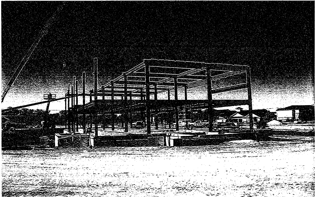
Erection of steel and placement of floor slab on October 20, 2010
