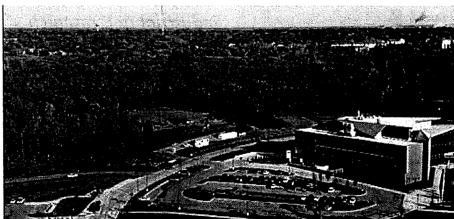
Construction of the Lawrence-Douglas County Bioscience Authority wet lab incubator began in October 2009. The complex will initially house eight to 11 companies and furnish 90 to 110 jobs.
