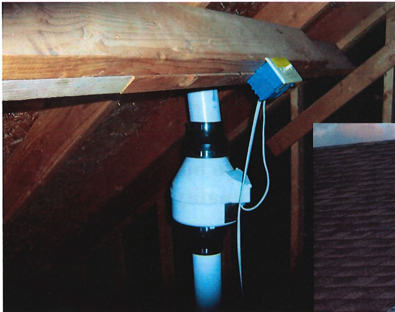
Attic installed radon fan
