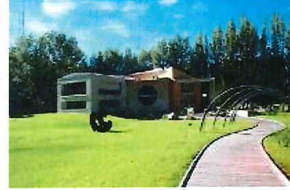
HQ & Visitor Center
