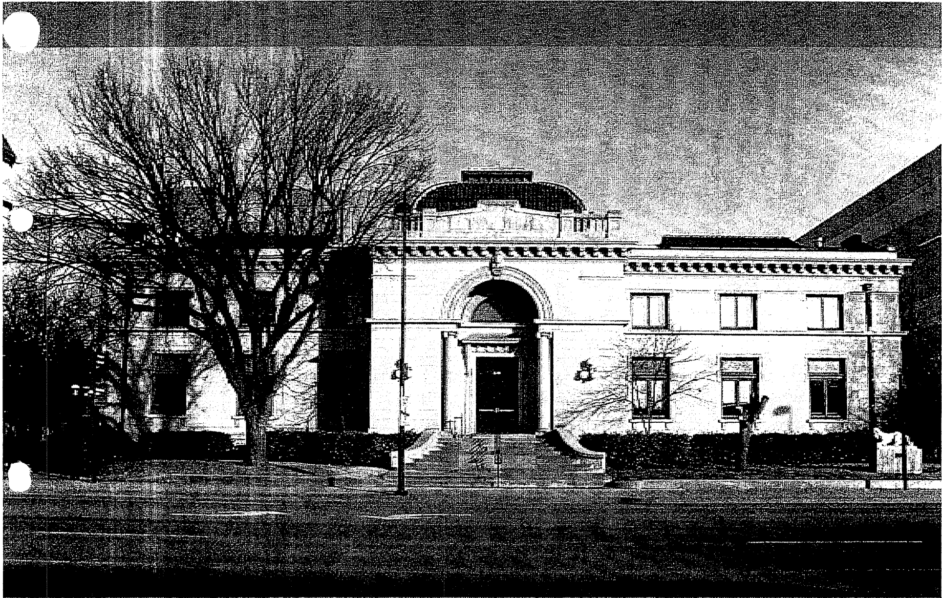
Carnegie Library - Fidelity Bank $5 M rehab
