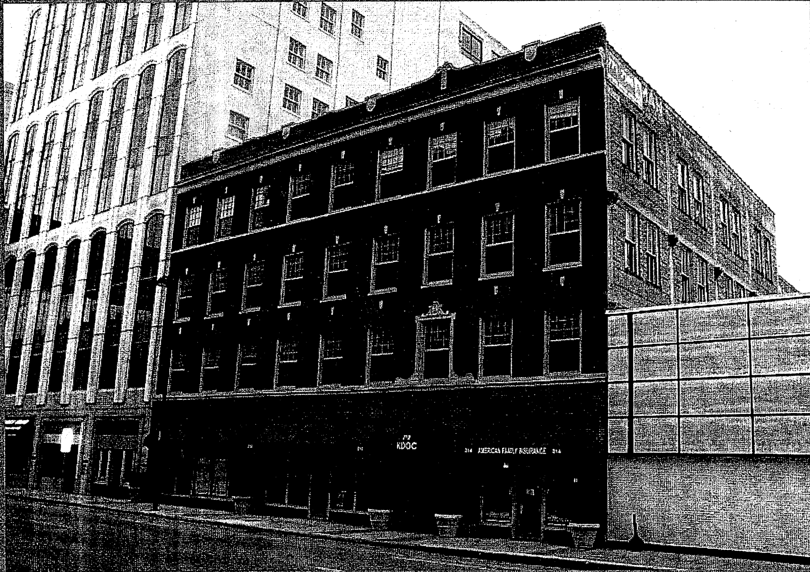
Kaufman Building $2 M storefront replacement, window repair and interior rehabilitation
