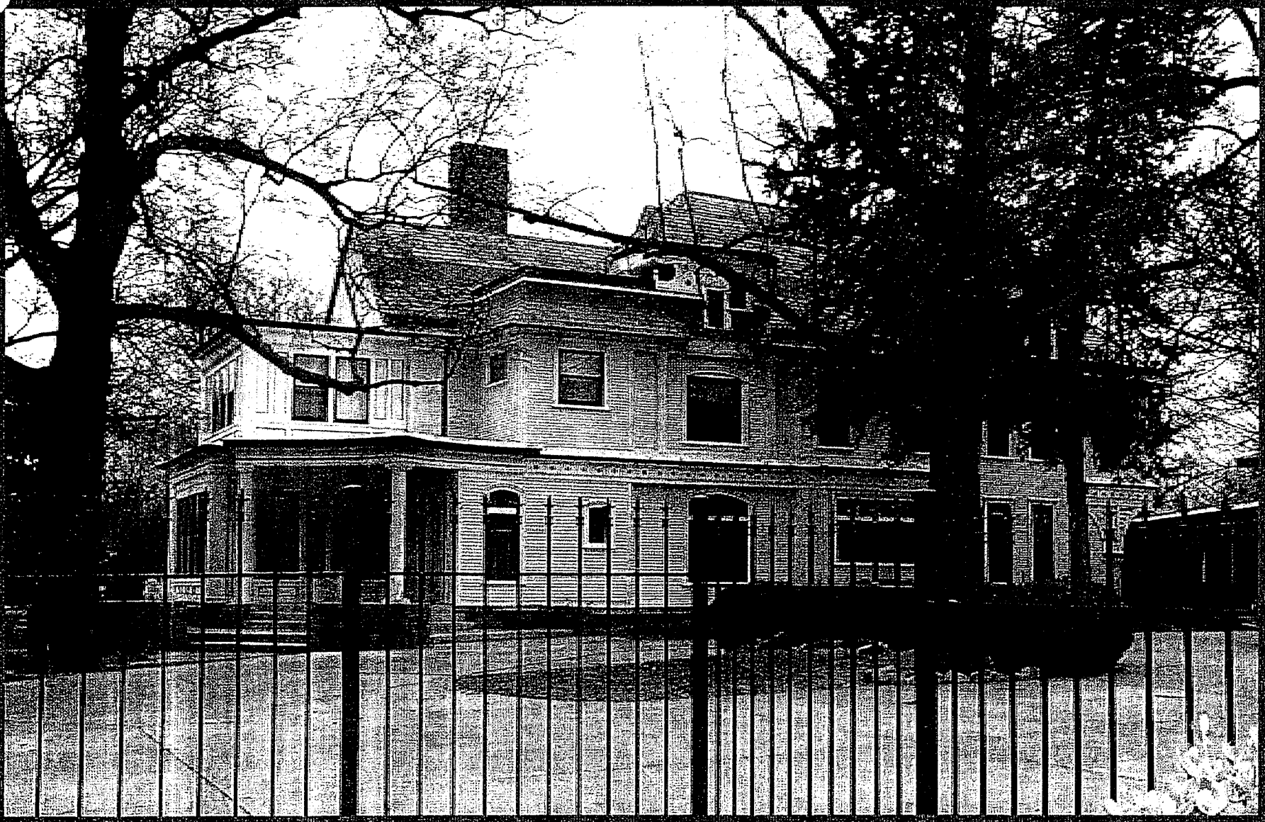
$400 K rehabilitation - LW Clapp House
