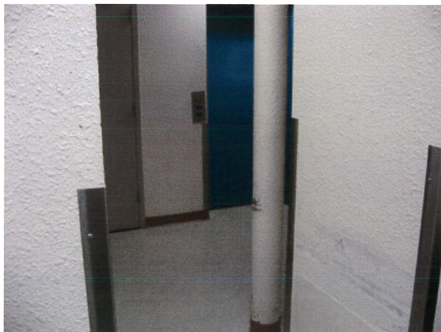
Exhibit F – Hallway Elevator Entrance Blind Spot (Camera Located Around Corner to the Right)
