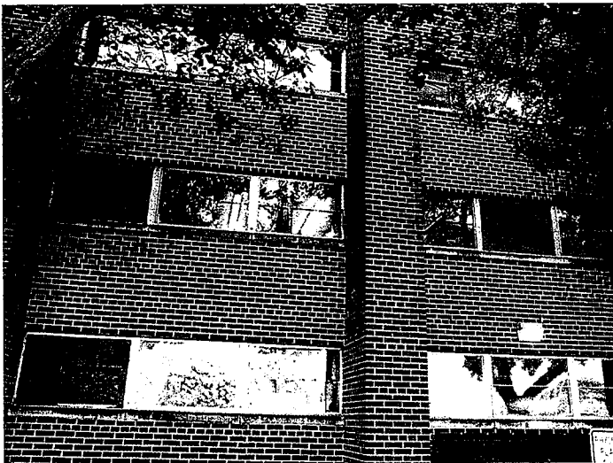
Single Pane Windows Multiple Locations
