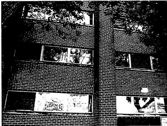
Single Pane Windows Multiple Locations
