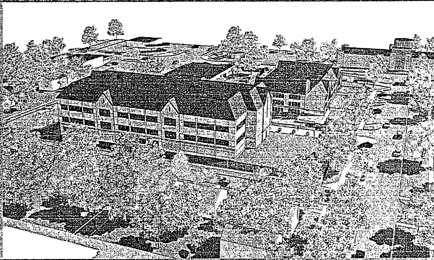
View From Northwest Corner
