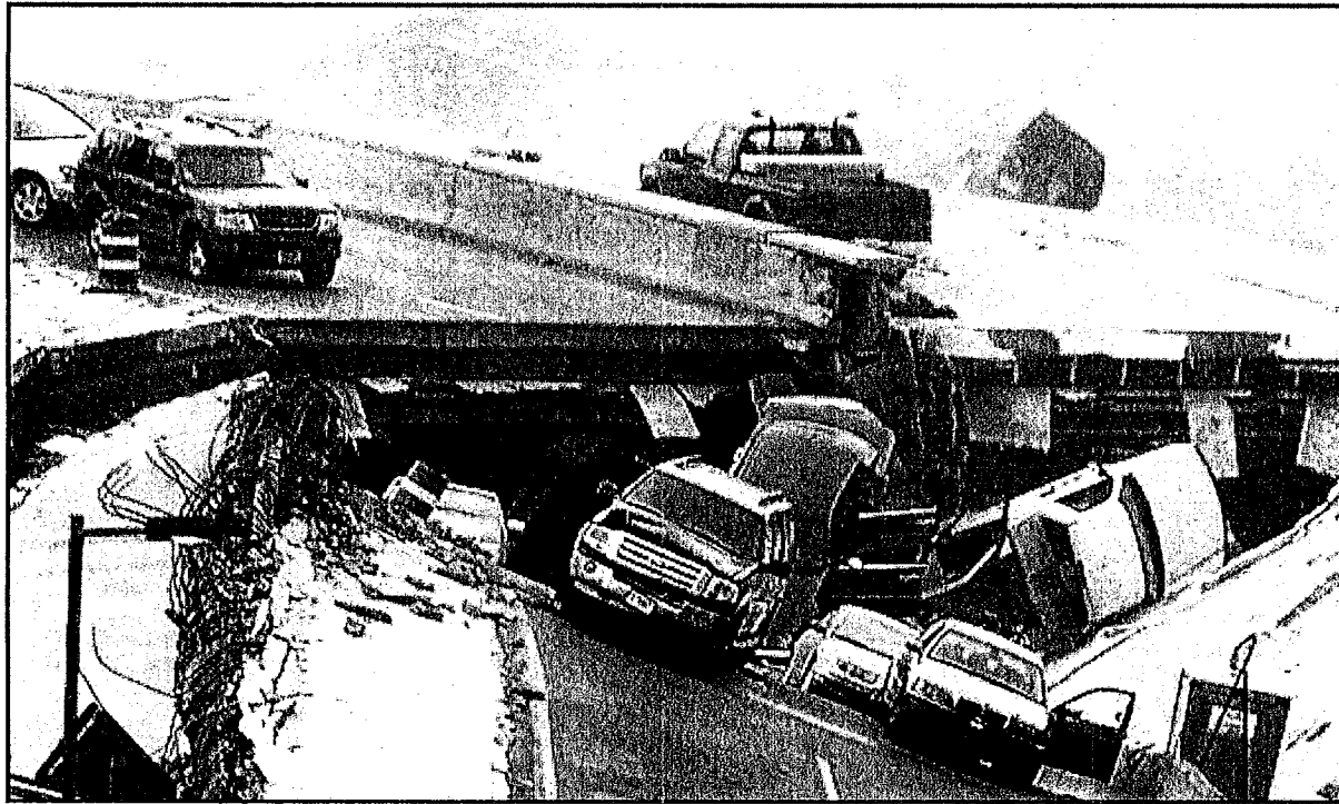
I35W Bridge Collapse – August 1, 2007, Minneapolis, MN
