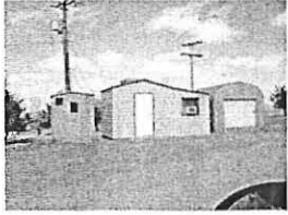
Water Tower Control Shed
