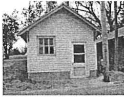
Walt Hall Steam Bldg
