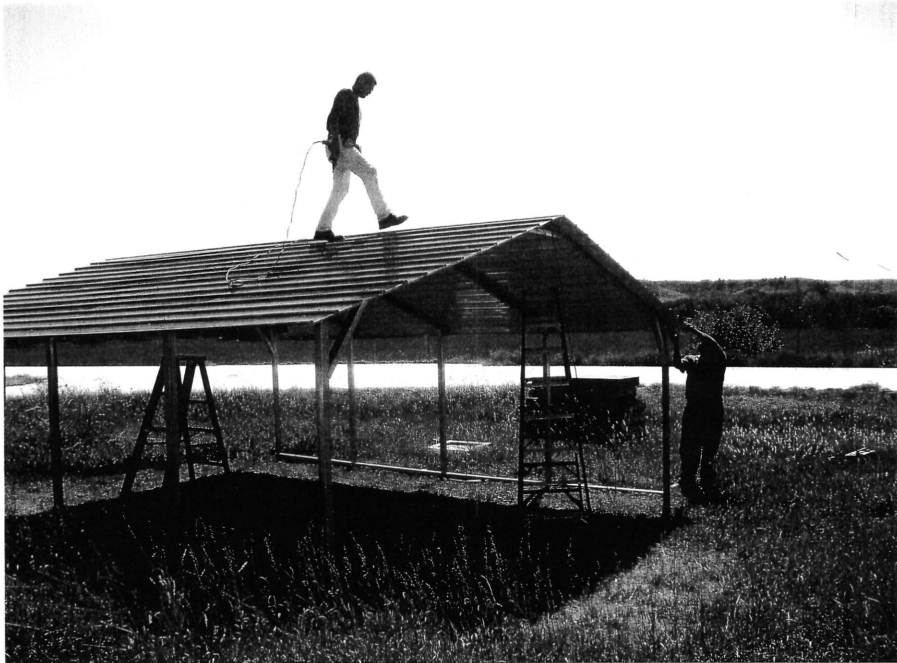
Erecting the Kill Creek Shelterhouse & Picnic Area for the Rediscovering Sod-House Days Heritage Backroad
