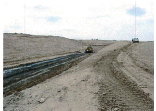
Construction, HorseThief Reservoir
