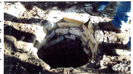
Abandoned Water Well
