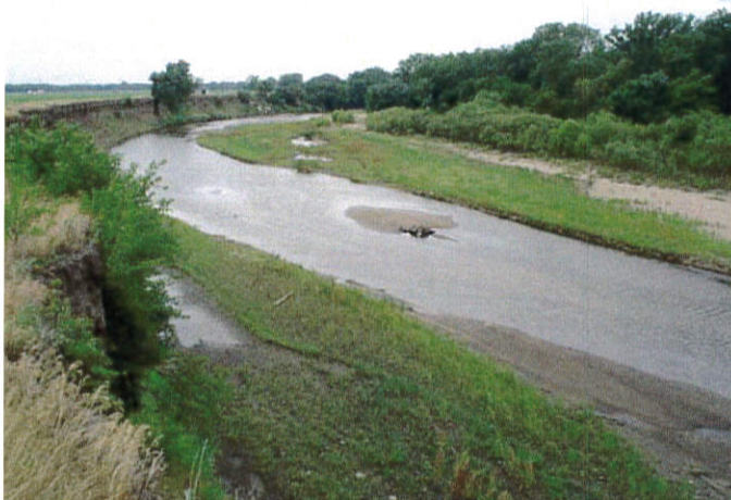
Streambank Stabilization - Before
