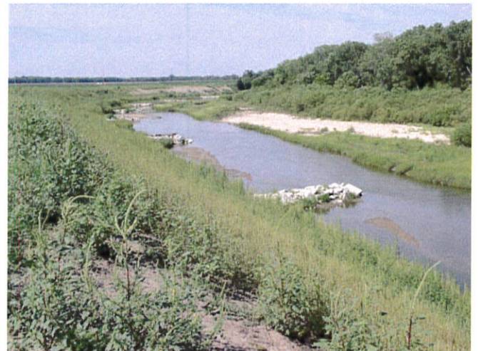
Streambank Stabilization - After
