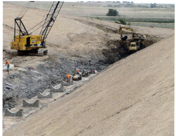
HorseThief: Principal Spillway Footing
