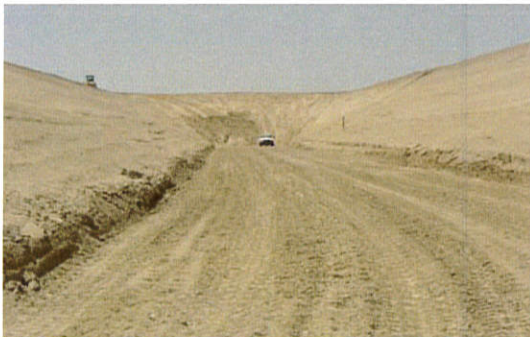
HorseThief: Core Trench
