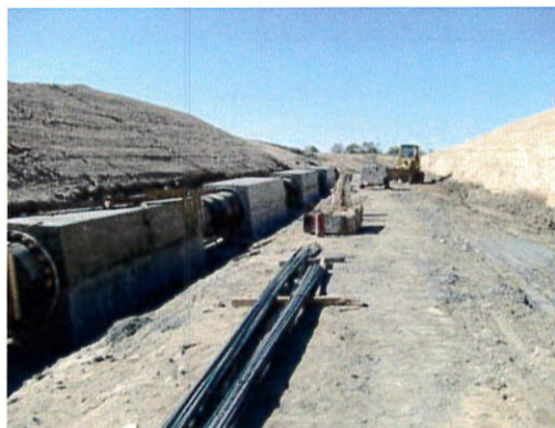
Principal Spillway Installation HorseThief Reservoir
