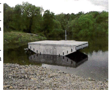
Critzer Dam First Filling May, 2007
