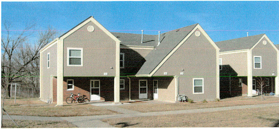
Rehabilitated Units. One to three bedrooms, $325 to $520 per month
