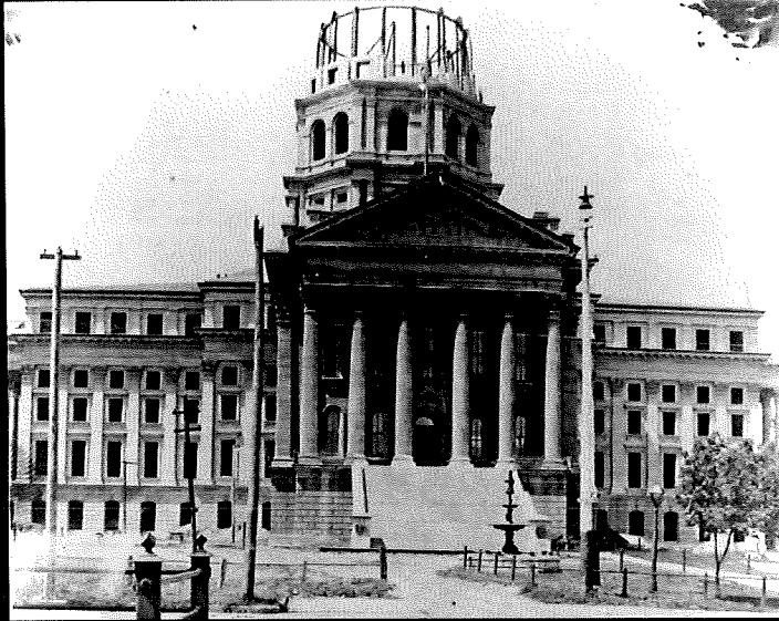
Dome Under Construction
