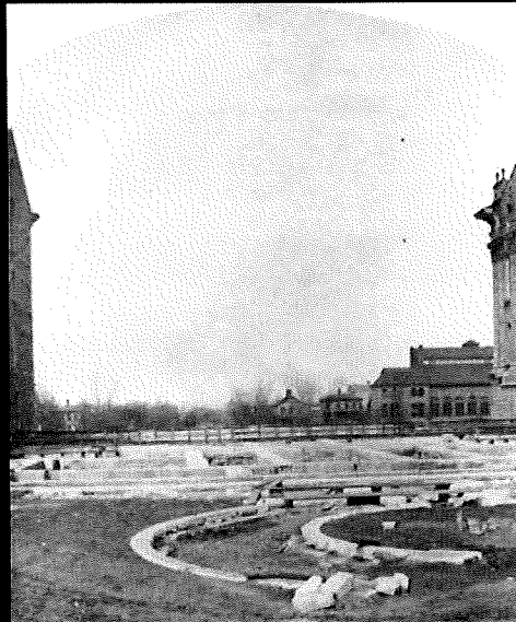
North & South Wing Construction Begins 1887
