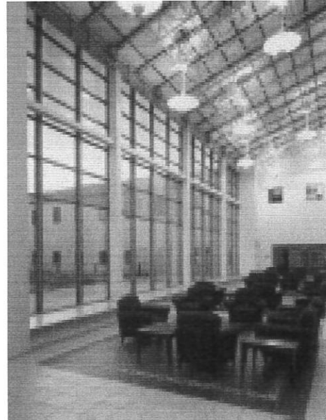
The first U.S. application of insulated architectural PV glazing was installed at the University of Wisconsin-Green Bay. The system, designed by Solar Design Associates, provides daylighting, cooling load mitigation, and solar-generated power to the new student center.
