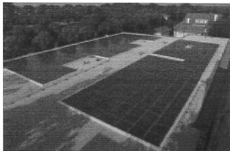
The Winston School, in Dallas, Texas, houses a 57-kW roof-mounted photovoltaic system. Data generated by the photovoltaic system is incorporated into the school's educational curriculum.
