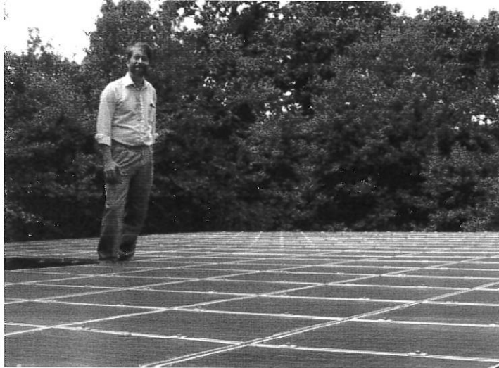
Steven Strong, President of Solar Design Associates, stands with the 10-kWp PV array his firm designed to feed solar-generated power into the White House distribution system; it was completed this summer.
