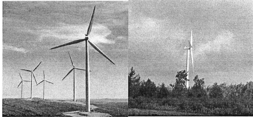
Blue Canyon Wind Farm 225 MW, near Lawton OK
