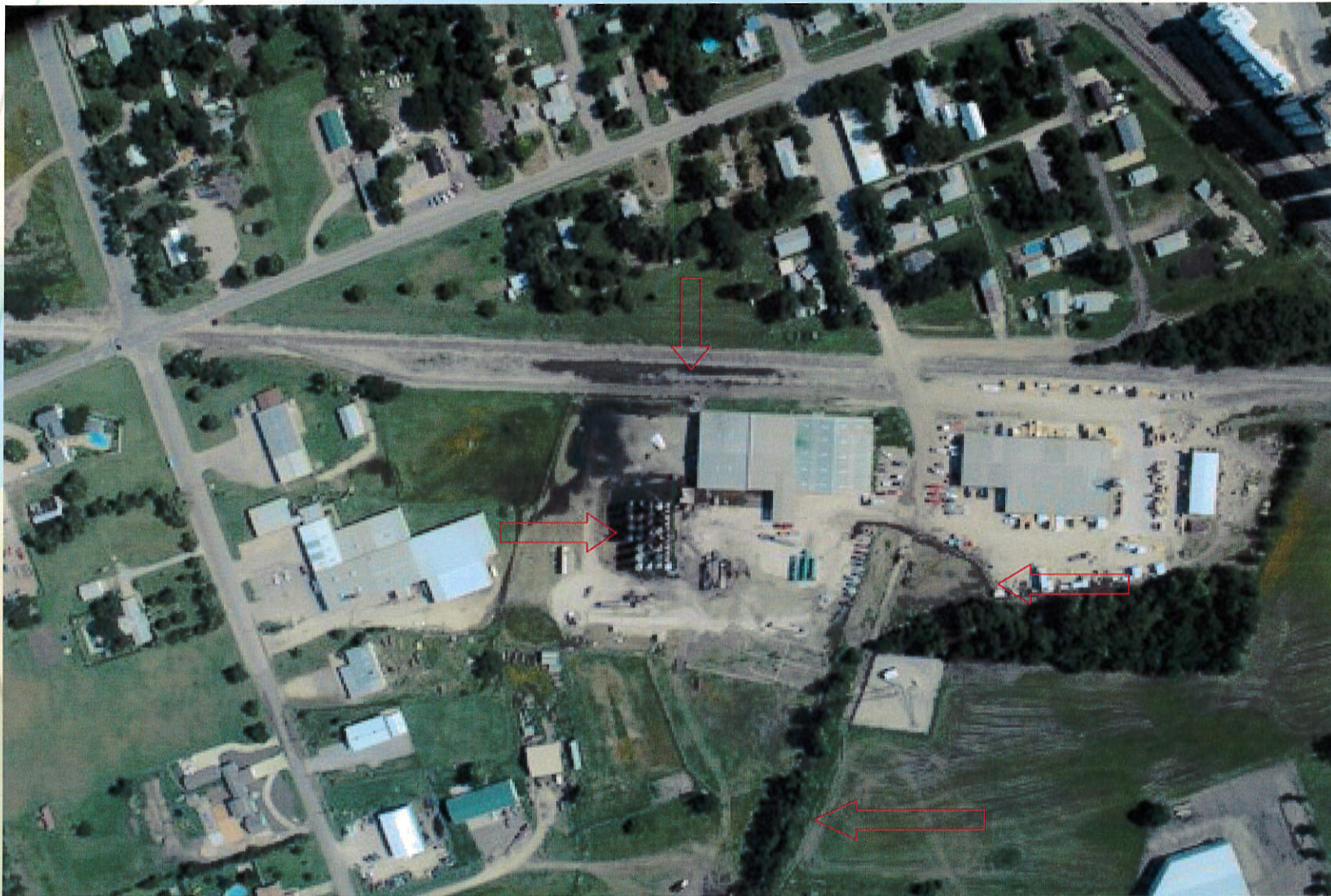
Various Chemicals, Fire Water and Foam Spread Over The Site.
