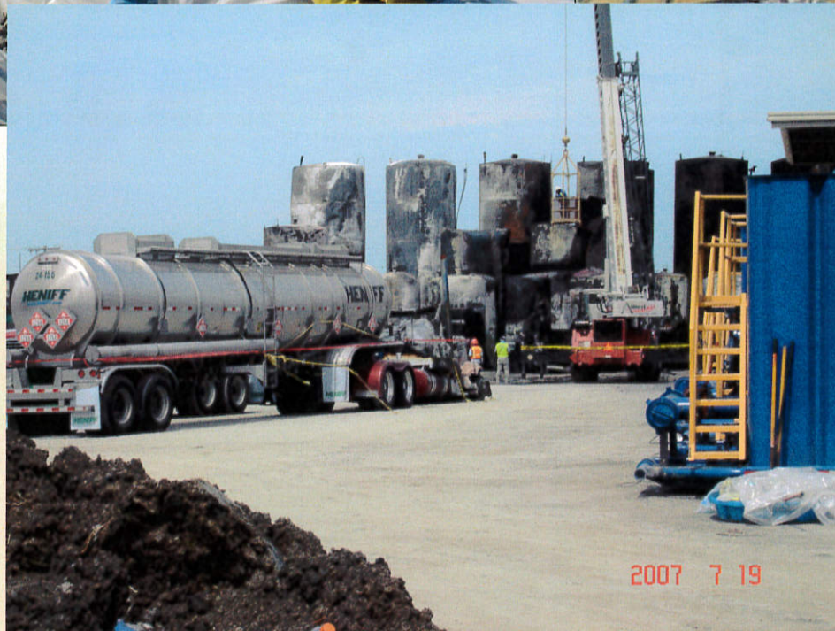
Tank Demolition, Off-site Soil Excavation and Characterization.
