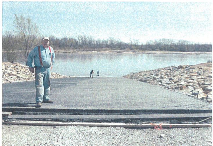
Boat Ramp Located on Western Property in Final Stages
