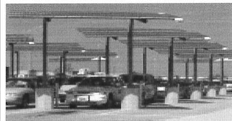
A ground-mounted PV array provides shading for the taxi stand at the Austin airport as part of Austin's Energy green pricing program.
