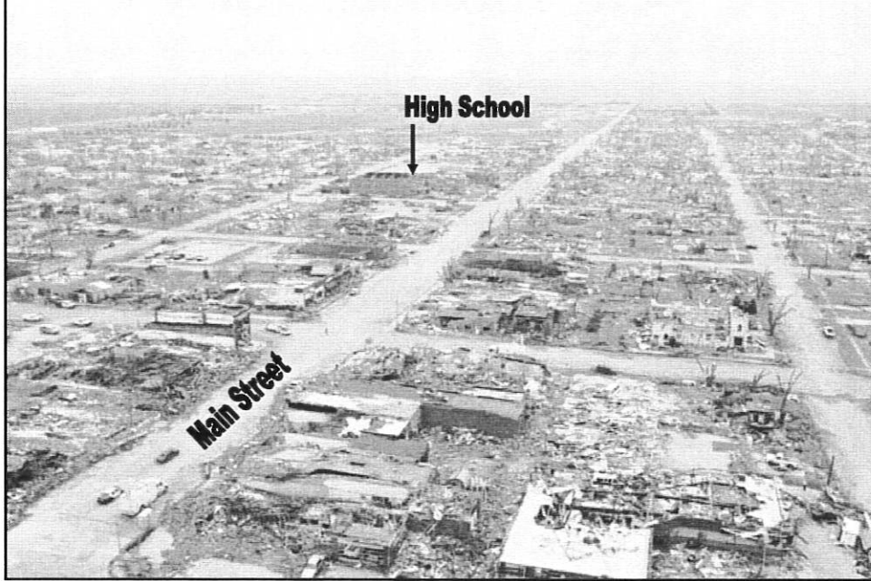
Aerial view of Greensburg looking south-east
