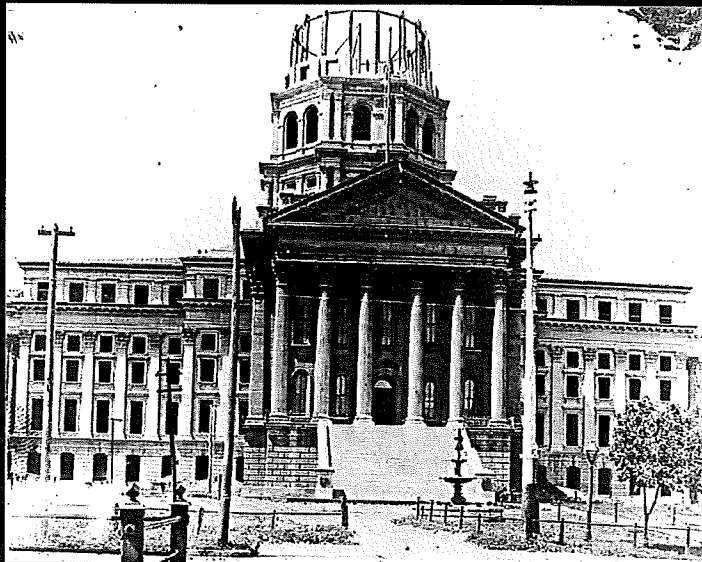
Dome Under Construction
