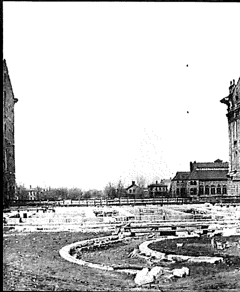
North & South Wing Construction Begins 1887
