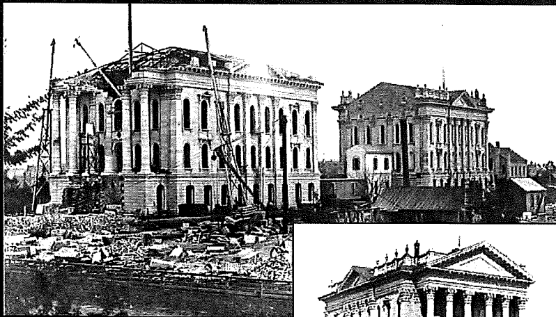
West Wing Construction 1879 - 1881
