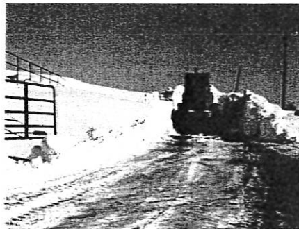
Clearance of trees, building wreckage, sand, mud, gravel, other disaster related material
