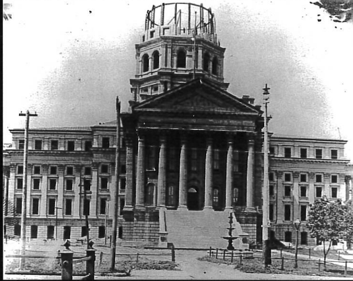
Dome Under Construction
