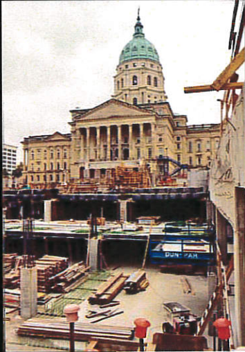
Parking Garage Under Construction
