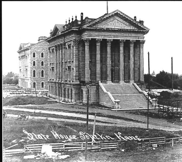
North & South Wing Construction Begins
