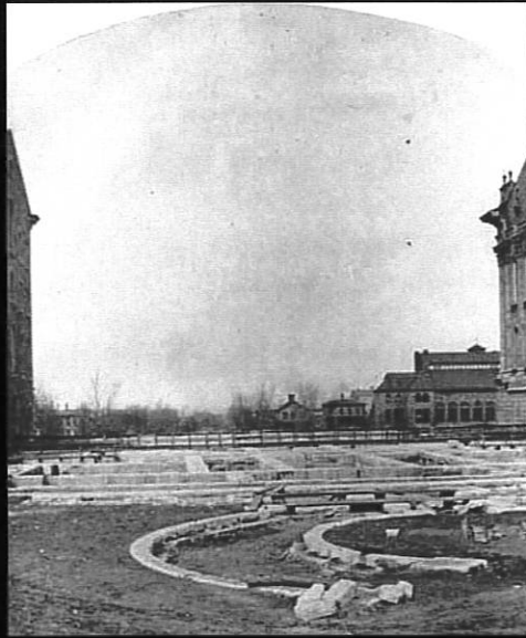
North & South Wing Construction Begins
