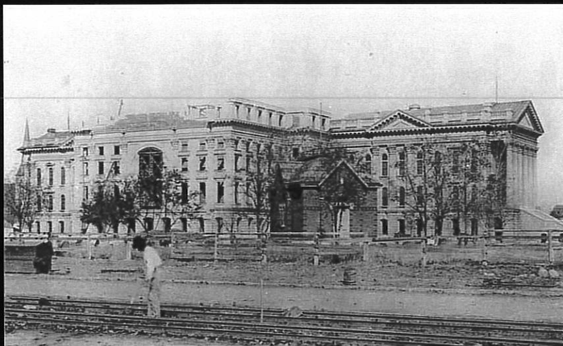
View of South Wing Under Construction
