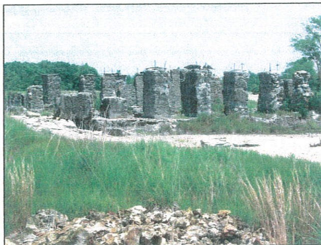
These old pillars stand watch over a wasteland that at one time provided a living to as many as 44,000 people.
