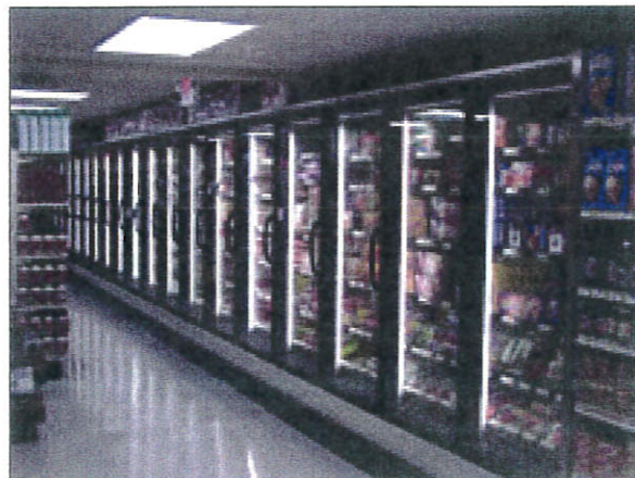
New energy efficient refrigeration units following installation.
