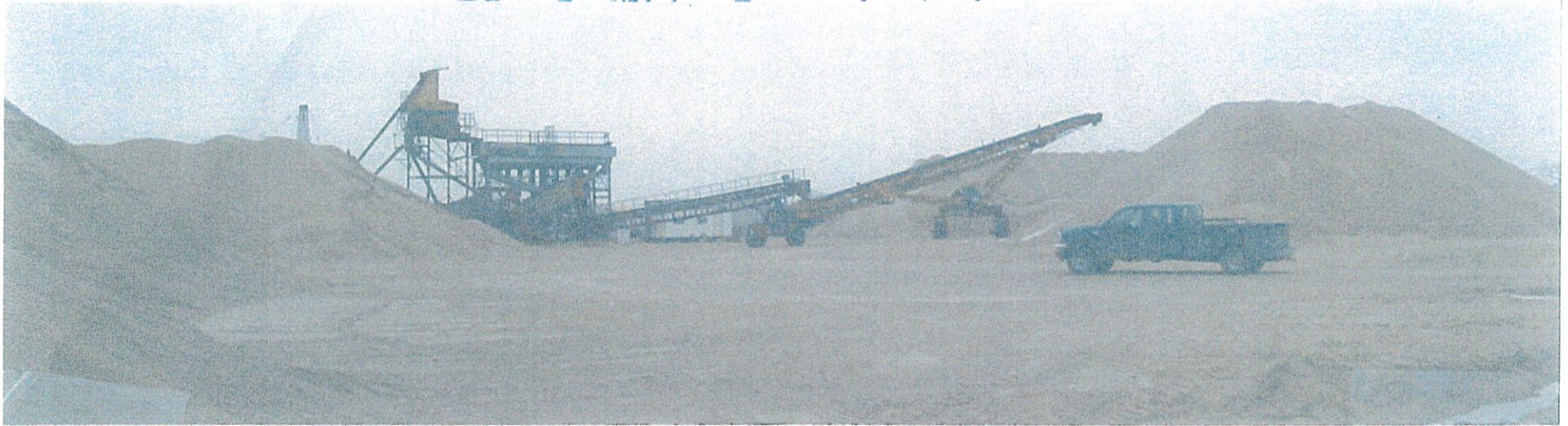
CONCORDIA SAND PLANT + STOCKPILES
