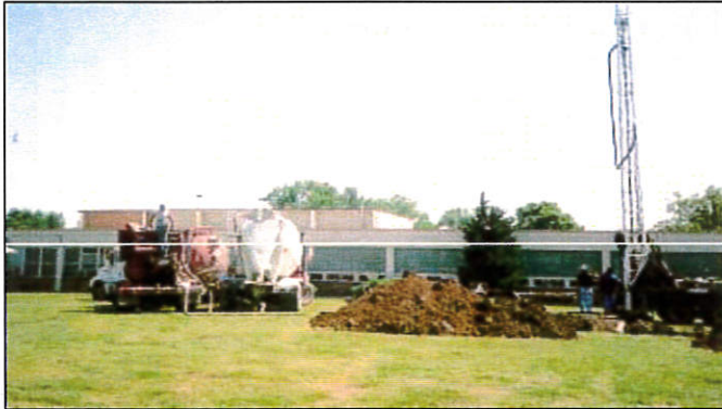
Well plugging at the Whittier School, Coffeyville
