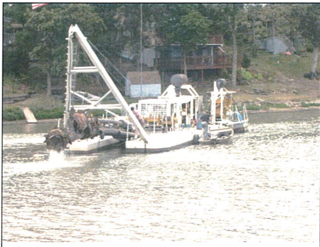
Sediment in Lake Dabinawa in Jefferson County was removed by the Masters Dredging Company, Inc., and pumped to settling, or material basins. The water was returned to the reservoir without the silt.
