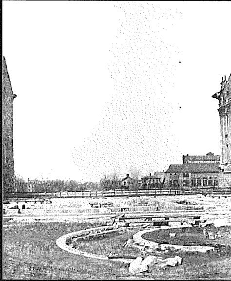
North & South Wing Construction Begins
