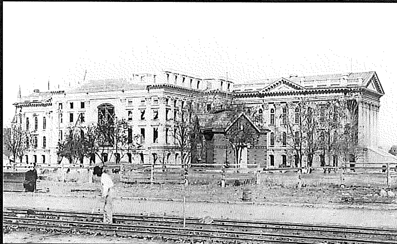
View of South Wing Under Construction
