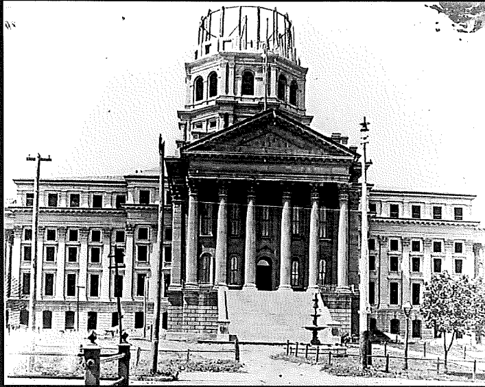
Dome Under Construction
