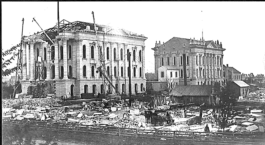
West Wing Construction
