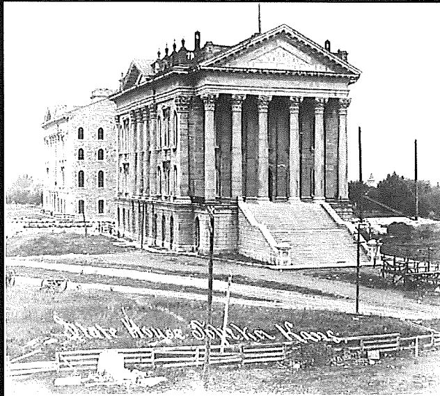
North & South Wing Construction Begins
