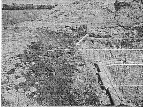
ABANDONED WELL FOUND DURING EXCAVATION FOR HOUSE, BUTLER CO.
