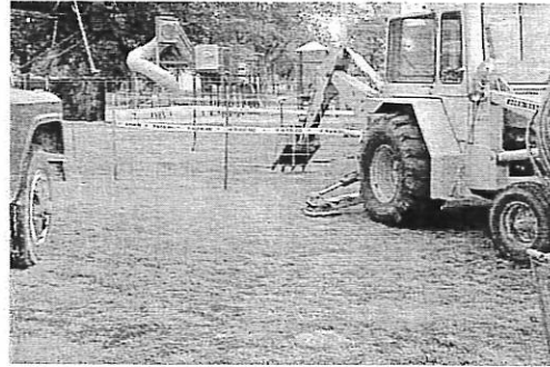
ABANDONED WELL IN SCHOOL YARD LOST SPRINGS, MARION CO.
