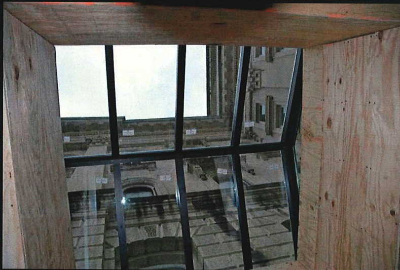
Ground Level Corridor with Skylights
