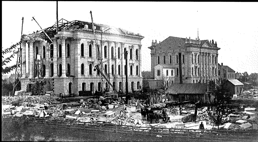
West Wing Construction
