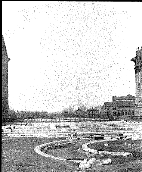
North & South Wing Construction Begins
