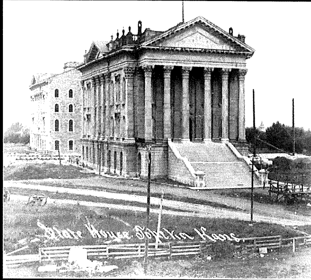
North & South Wing Construction Begins
