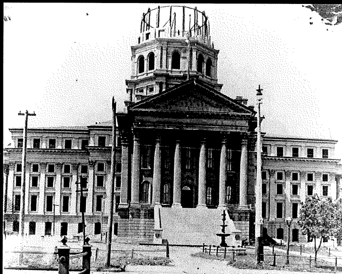
Dome Under Construction
