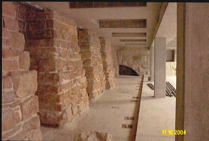
Ground Level Corridor with Skylights
