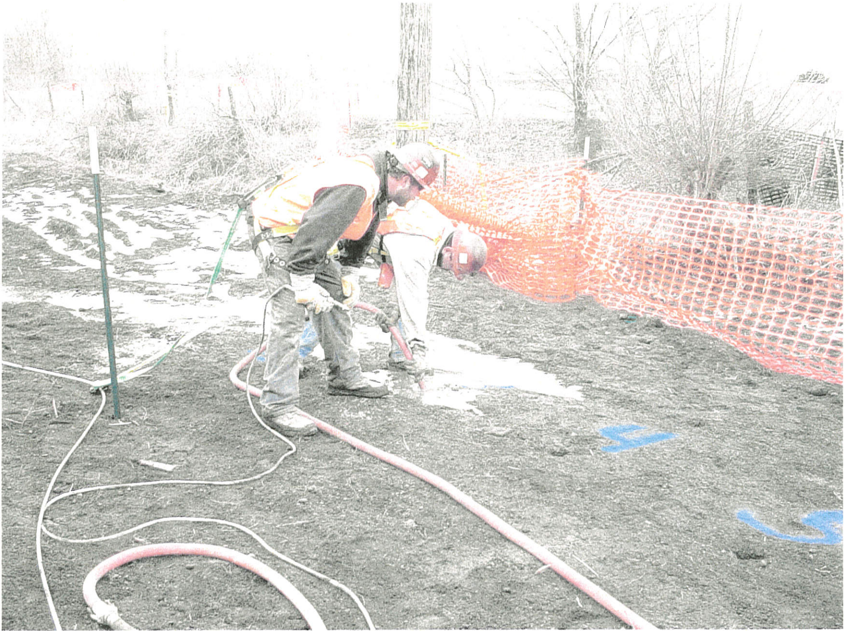
North Wall of Sinkhole Grouting
