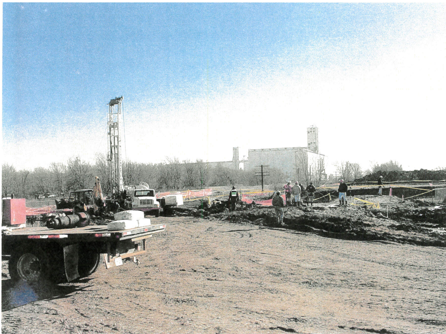
Drill Rig for Test Hole #2
