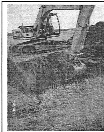
Excavating Abandoned Well Kingman Co.
