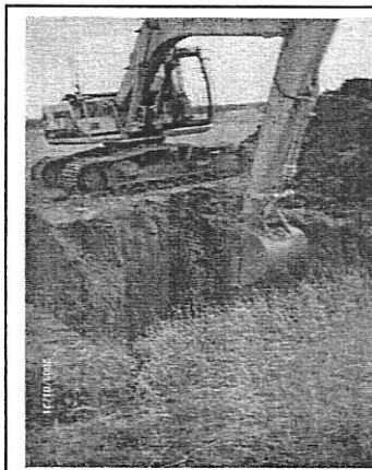
Excavating Abandoned Well Kingman Co.
