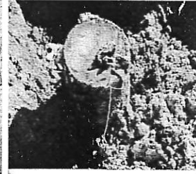
Abandoned Gas Well, Wyandotte Co. Venting Gas and Saltwater
