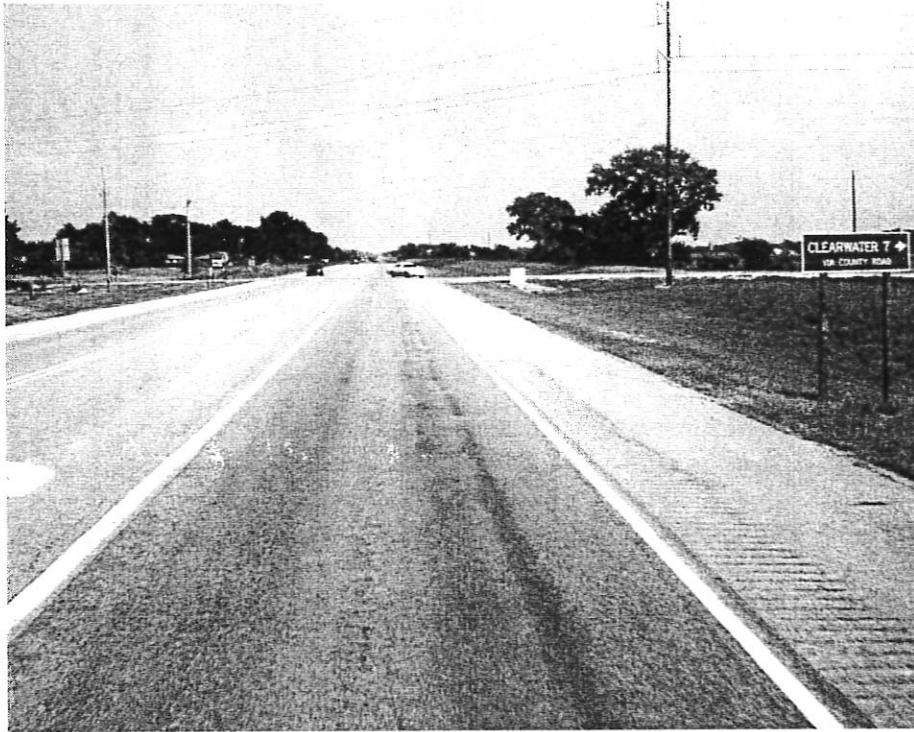
K-42, Eastbound at a County Road "Clearwater 7, Right Arrow, Via County Road"
