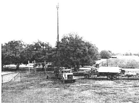
Abandoned Well in Schoolyard Lost Springs, KS
