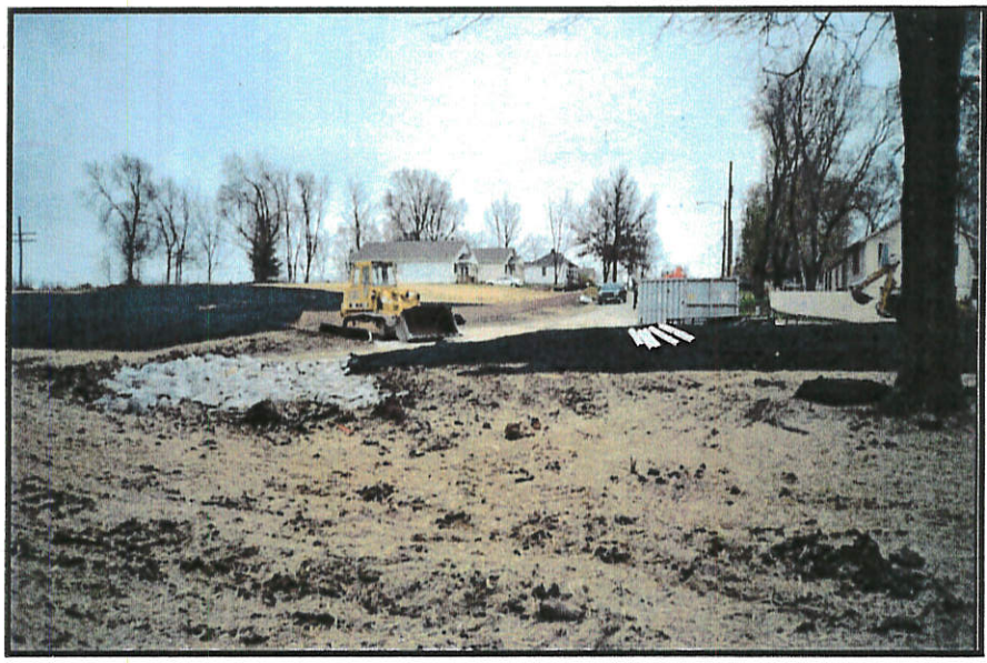
A cap was constructed with clean soil, an Enkamat cover, and vegetation as well as construction of a drainage ditch. Construction shown here is nearing completion.
