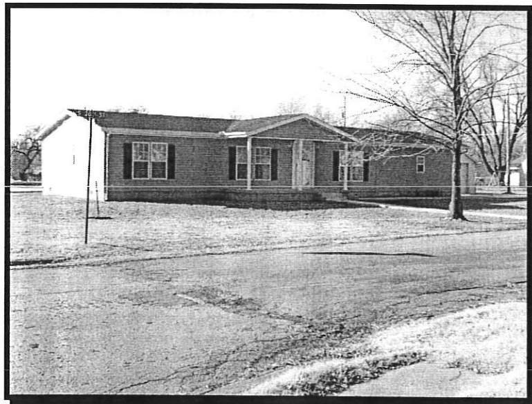
Manufactured Home Used As A Replacement Home for A Family Who Lost Their Home in the Tornado of April, 2000
