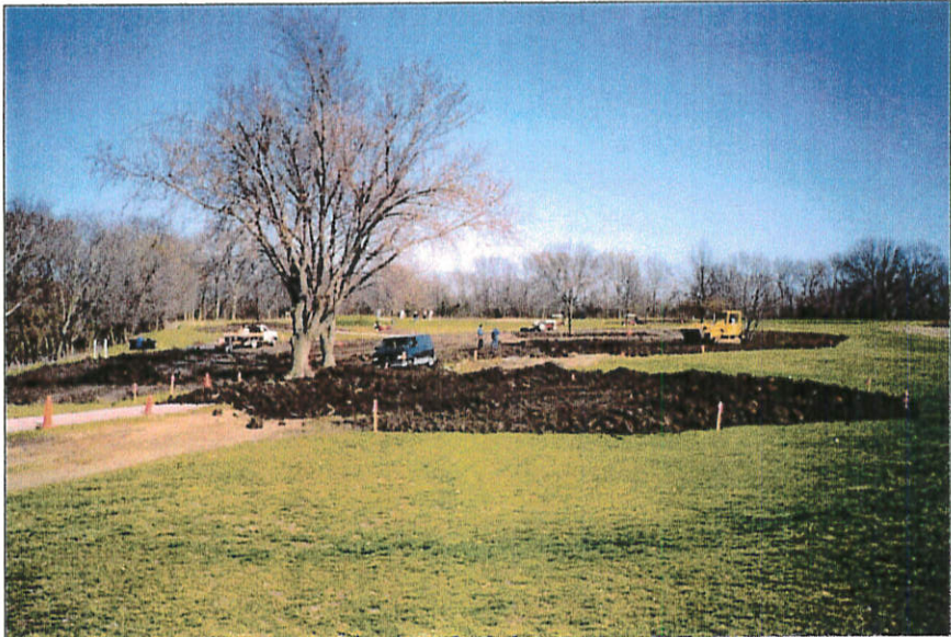
Cap construction over exposed battery landfill debris
