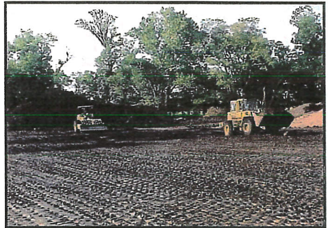
Placement and compaction of clay cap.
