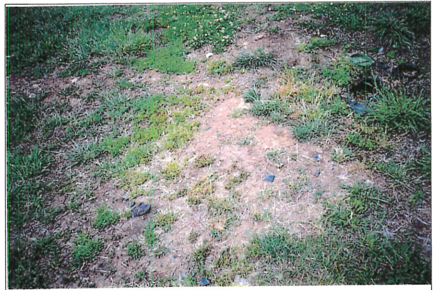
Exposure of battery debris following erosion of cap
