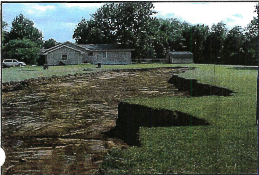
Excavated area of sludge impact on residential property.
