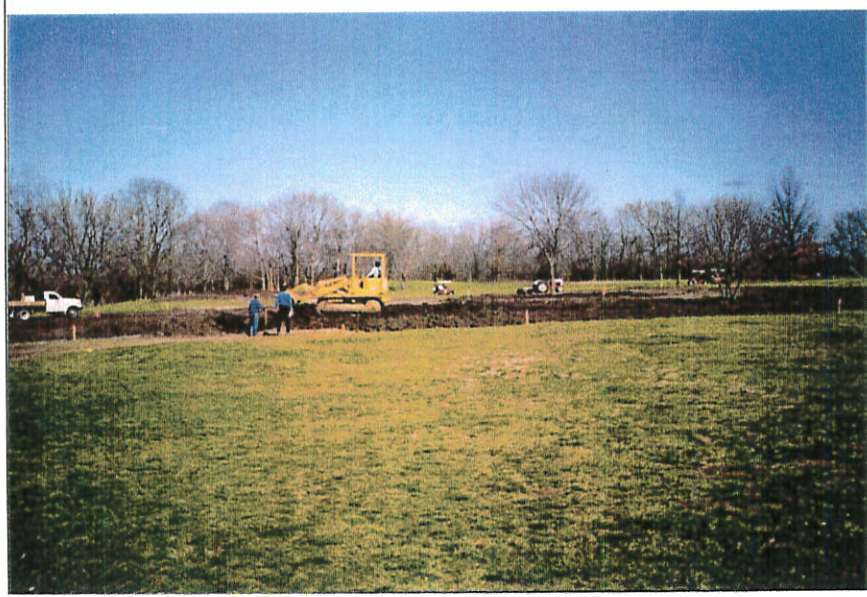
Cap construction over exposed battery landfill debris
