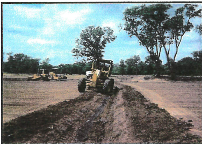
Construction of drainage swale.
