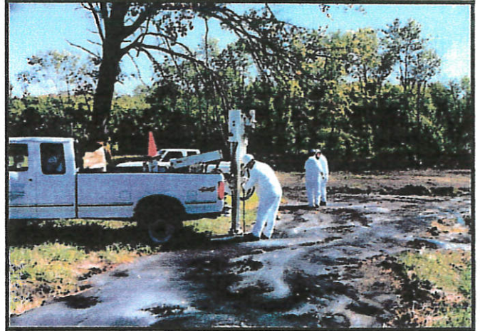
Sampling and characterization of sludge material.
